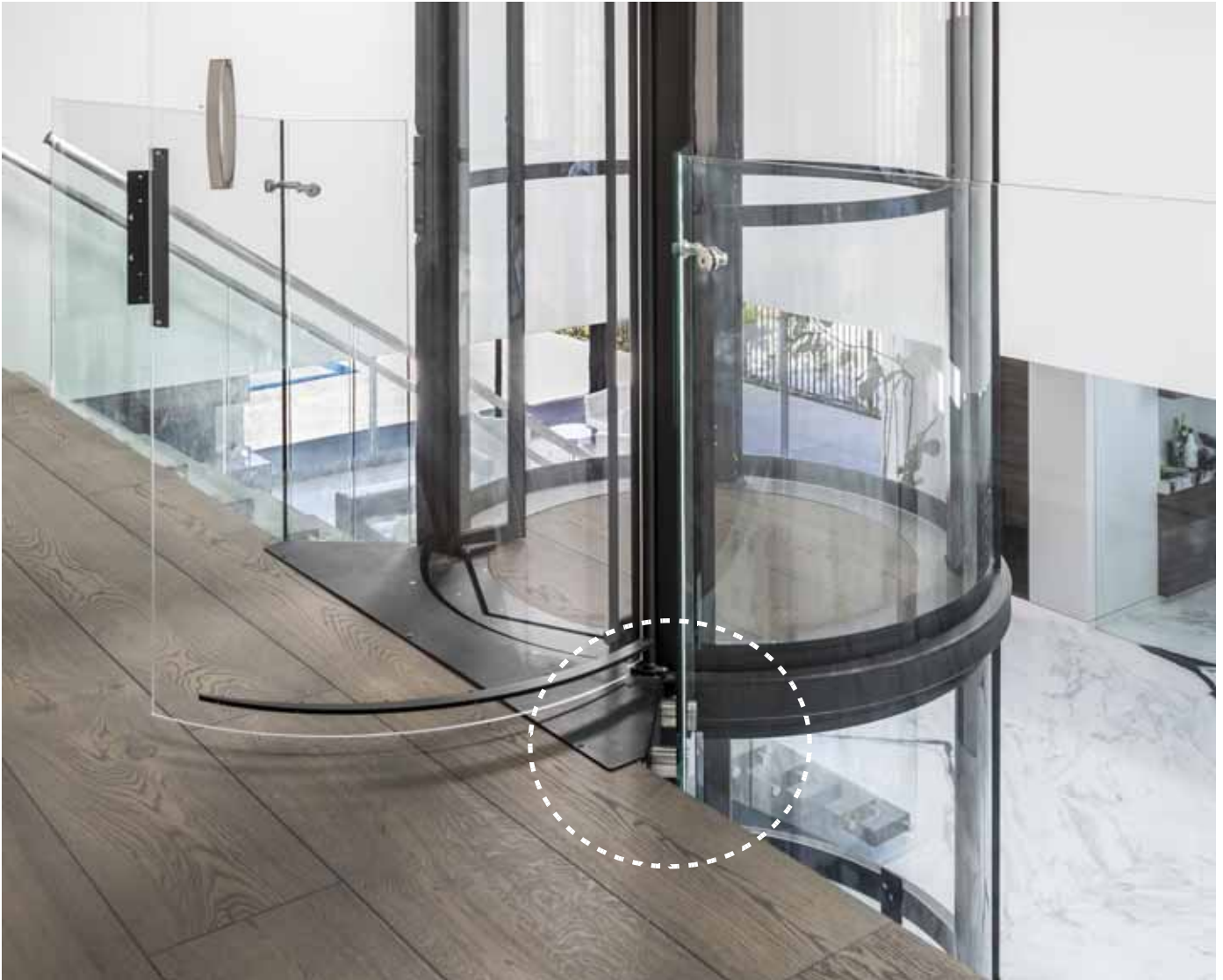
Figure 43: Balcony plate and handrail information (RGL)
