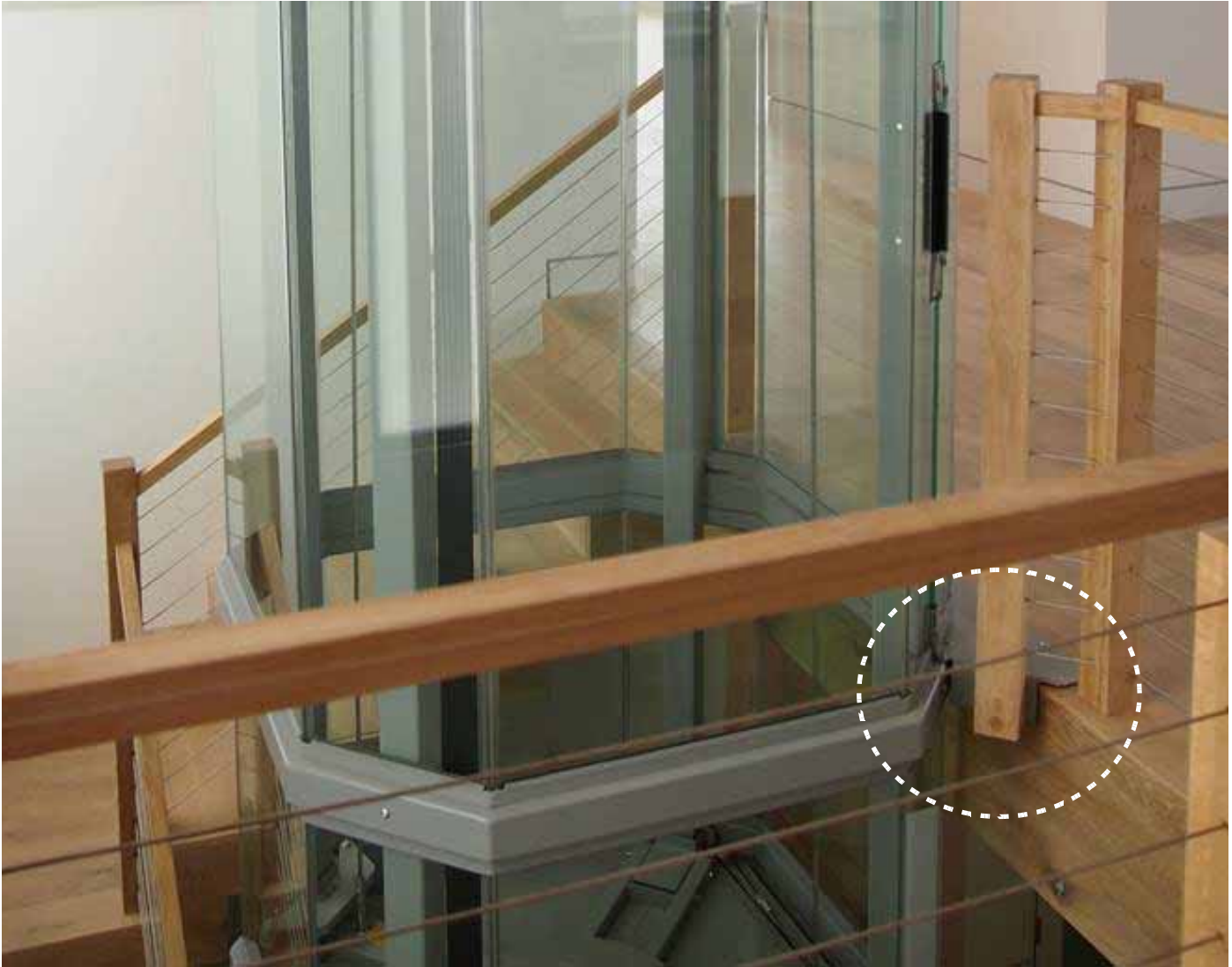
Figure 33: Balcony plate and handrail information (OGM, type 2)
