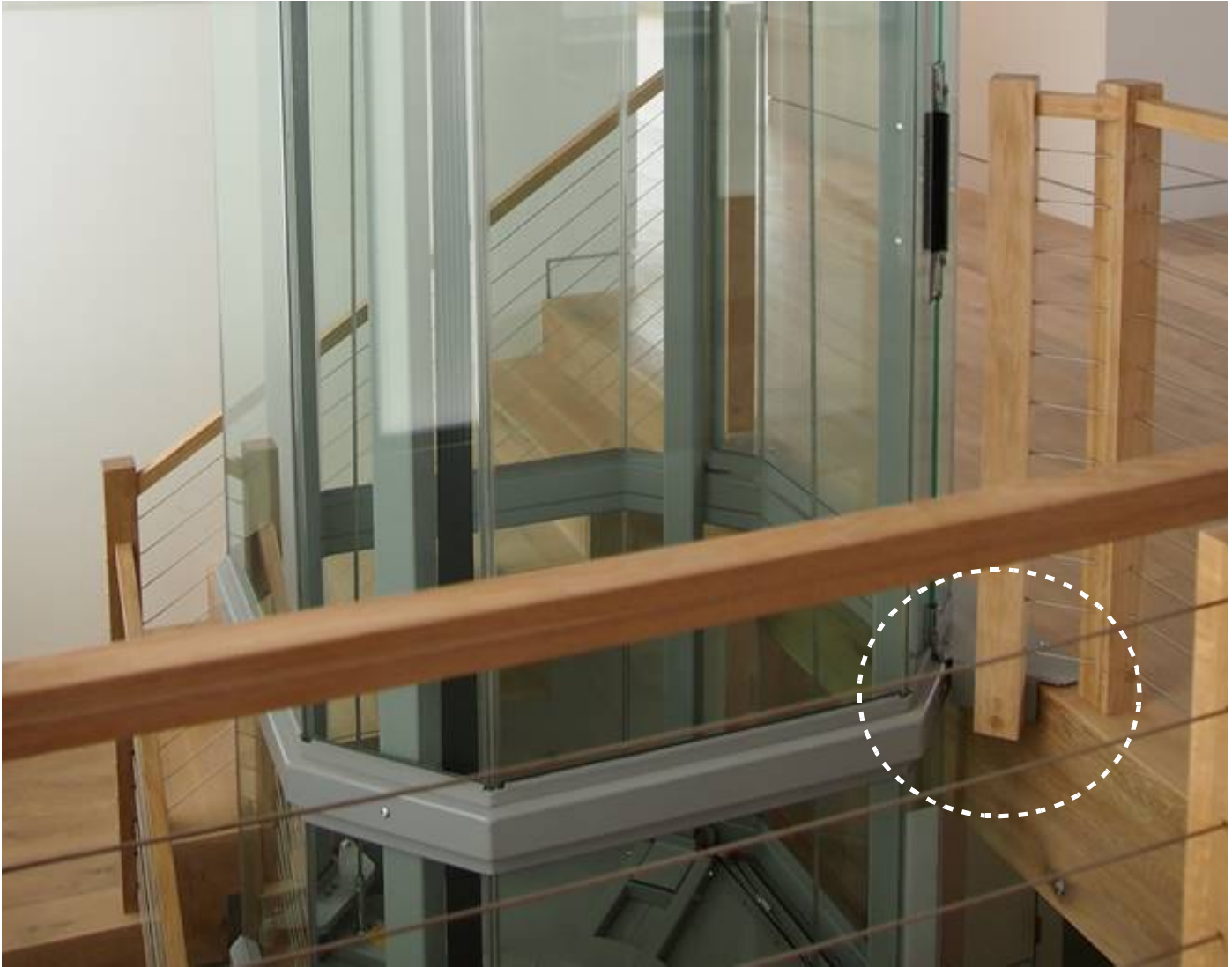
Figure 23: Balcony plate and handrail information - octagonal acrylic (OAM) type 1 shown
